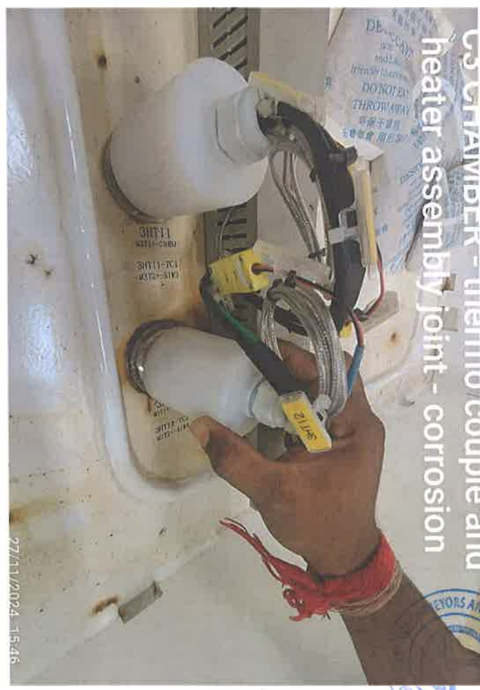
C3 CHAMBER - HEATING WIRE CABLE TRAY - CORRODED
